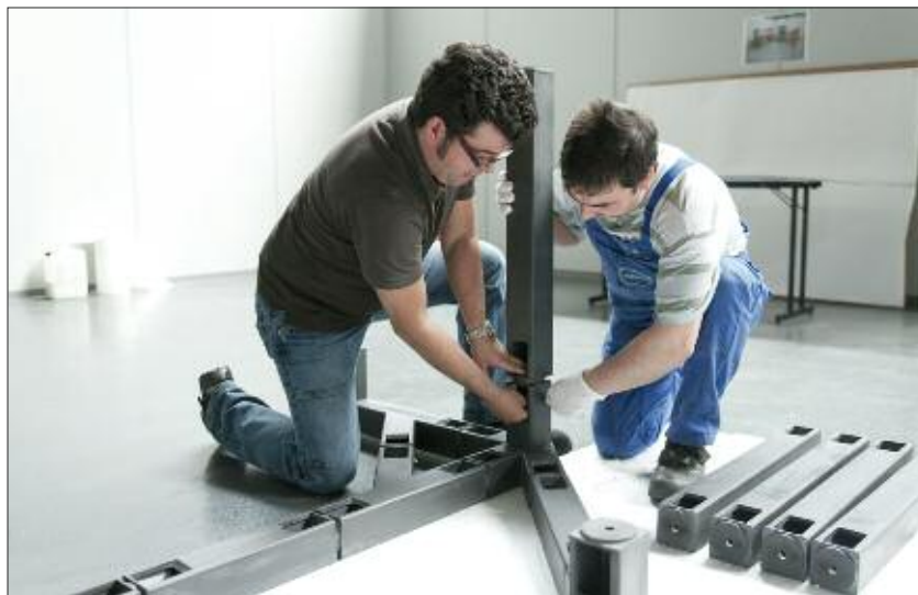
Fig. 1 Installation of truss elements (source: SCHUNK Ingenieurkeramik)
