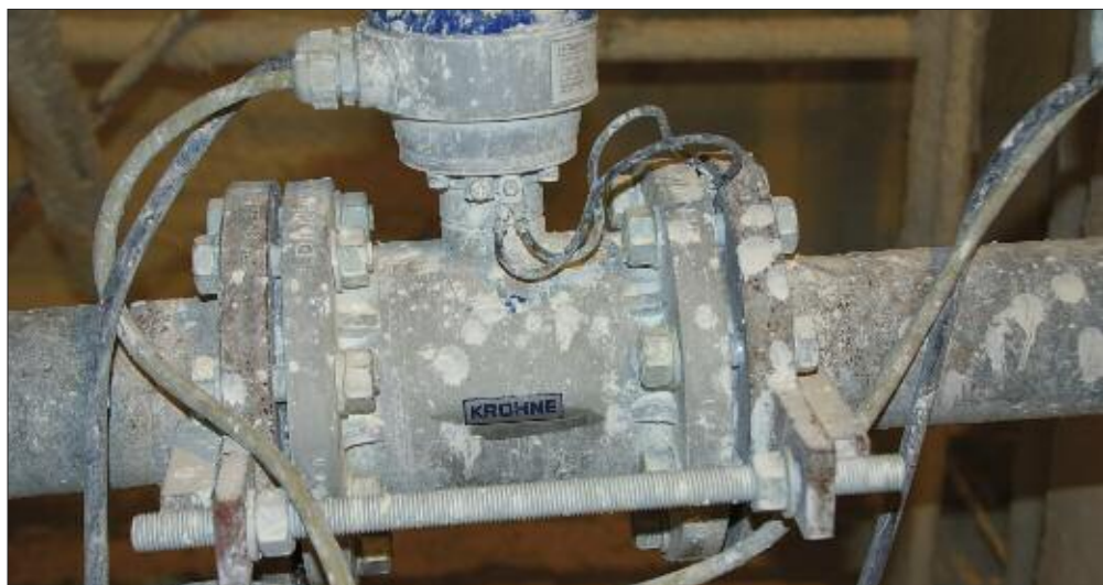
Fig. 11 OPTIFLUX 5300 measures highly abrasive magnesium hydroxide sludge
