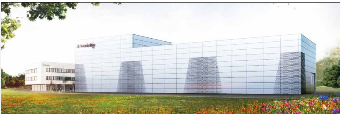
Fig. 3 The new fibre pilot plant building (Visualisation: KSG Architekten)
