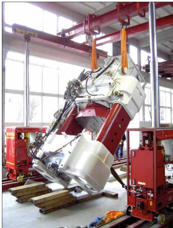
Fig. 6 Installation of ALPHA 1500
