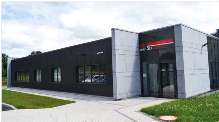
Fig. 1 New facility in Bonnac La Côte near Limoges
